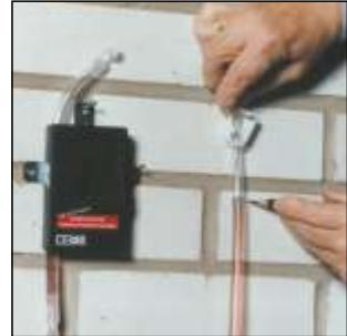
Do not fill the hose completely, 30 cm should remain free. Connect the hose to the appliance. Switch on the electronics. The control lamp lights up and indicates readiness for operation.
